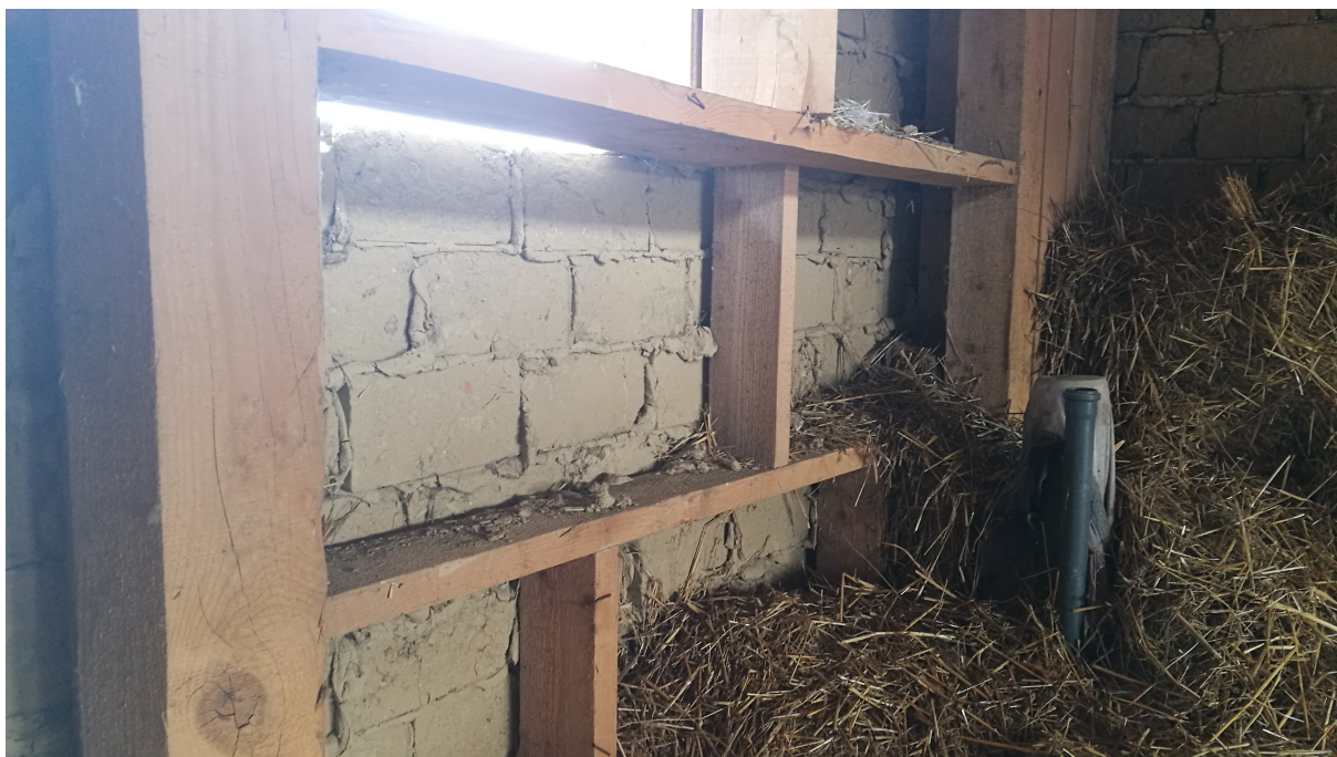
Figure 12 - Photography of the building wall structure
