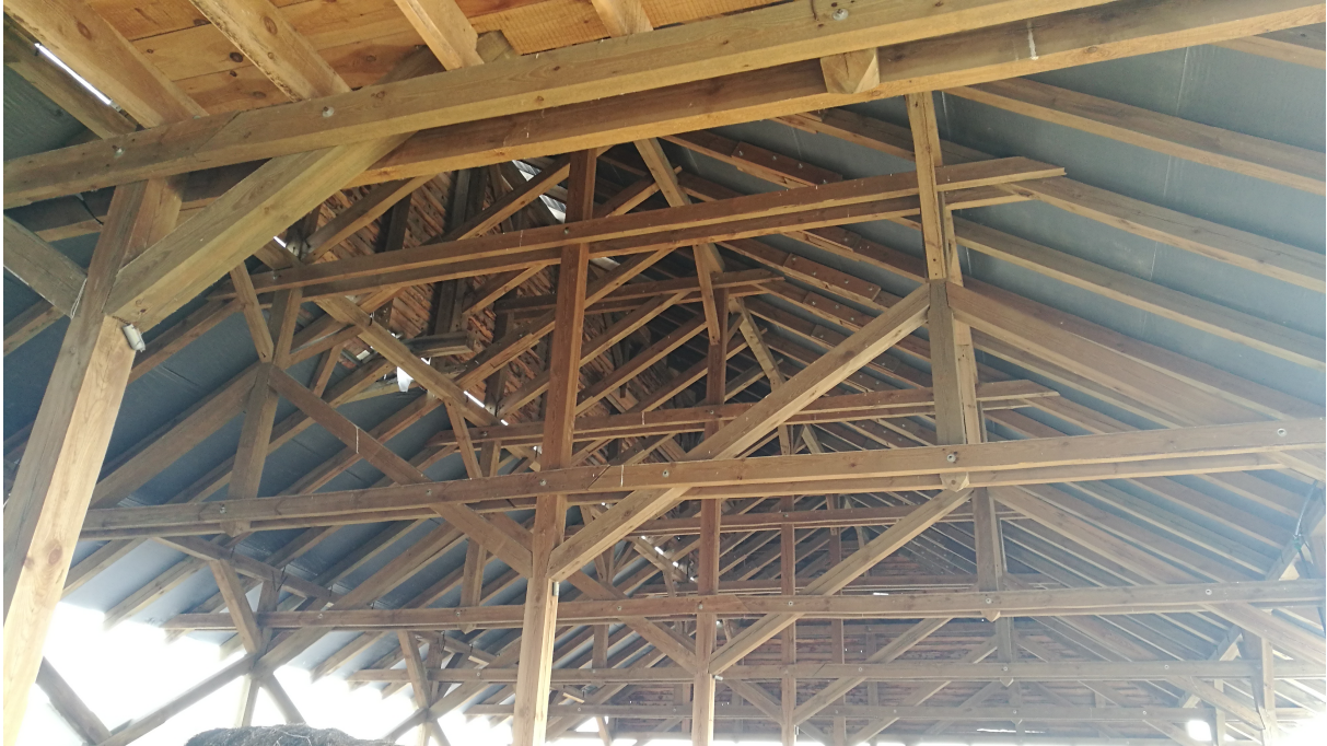
Figure 7 - Photograph of the wooden structure of a common eco-village building
