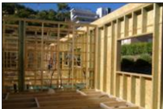
Figure 68. Construction with sandwich panels (wood, rockwool and wood). Source: Municipality of Serra (2011)
