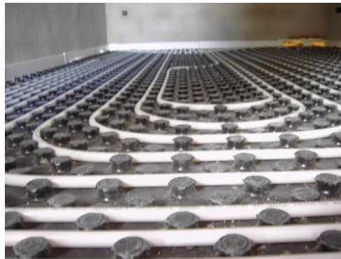
Figure 25. Underfloor heating. Source: Tecnoambient (n.d.)
