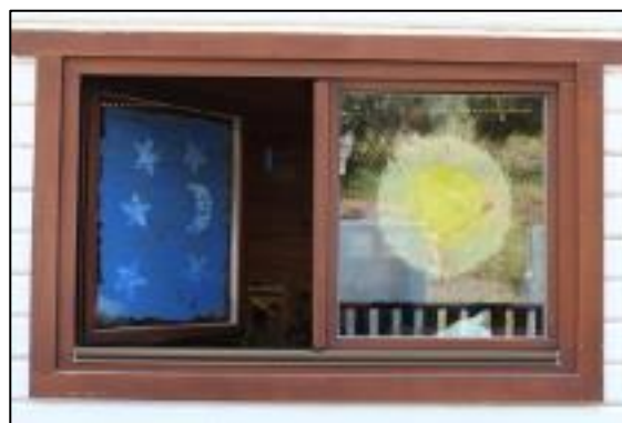
Figure 69. Insulated windows (double glazed). Source: Own elaboration
