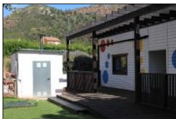
Figure 61. Boiler room. Source: Own elaboration
